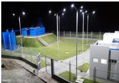
Potable water Plant Gualmatán, Nariño
