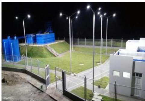
Potable water plant Gualmatán, Nariño
