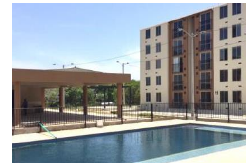
Parques de Bolívar housing project Santa Marta, Magdalena
