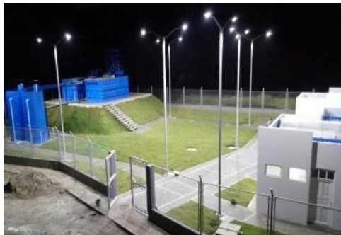
Potable Water Plant Gualmatán, Nariño
