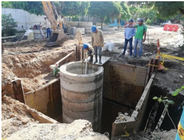
Installation of sewer networks.
