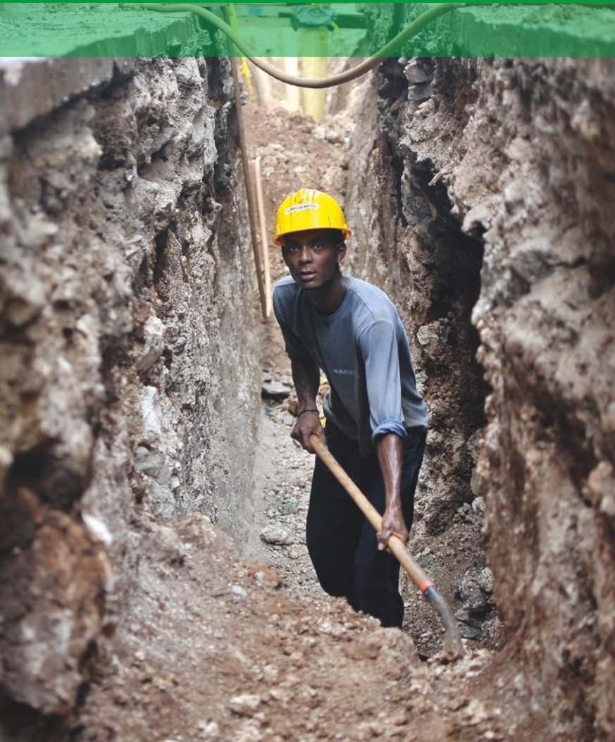
Renovation of San Andres Water System
