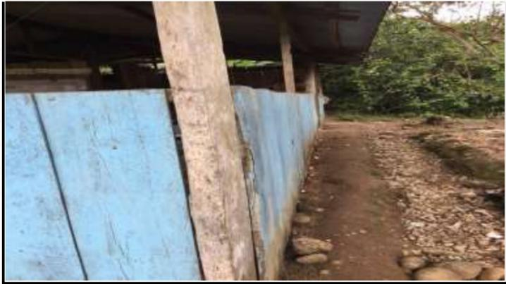
DETALLE DE MUROS EN MADERA
