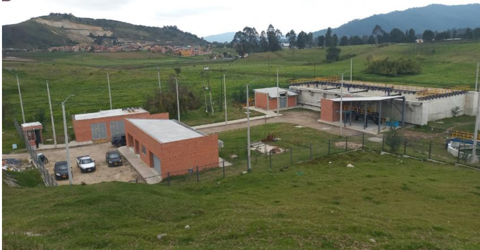
Illustration No. 33: General view of the constructed WWTP – Jan 2024, Facatativá
