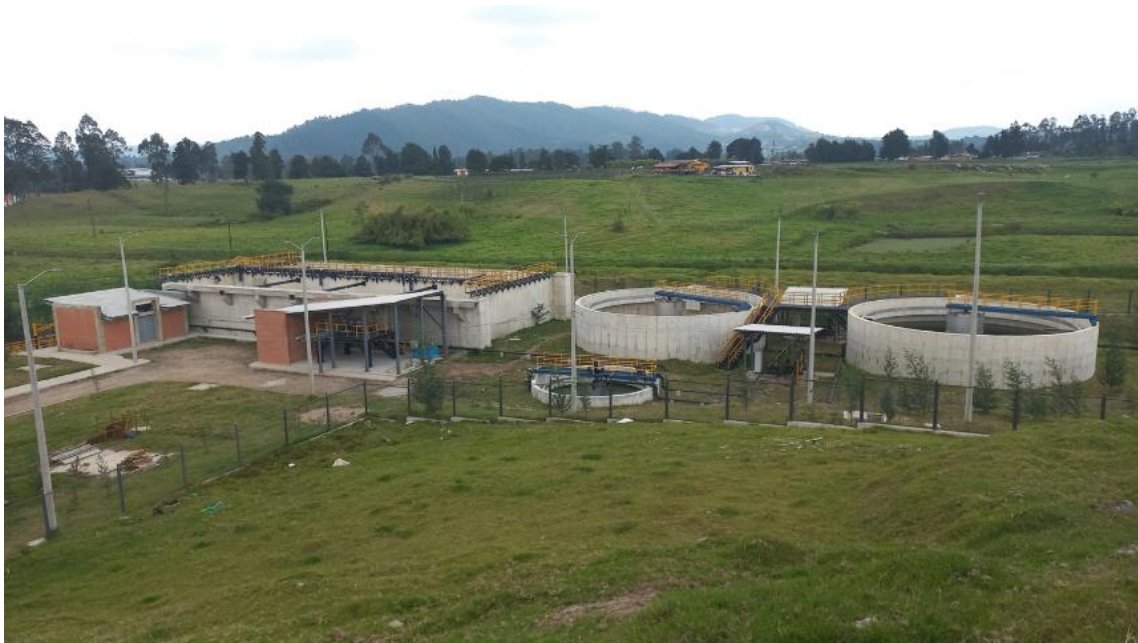
Illustration No. 33: General view of the constructed WWTP – Jan 2024, Facatativá
