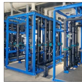
Racks for reverse osmosis and ultrafiltration.
