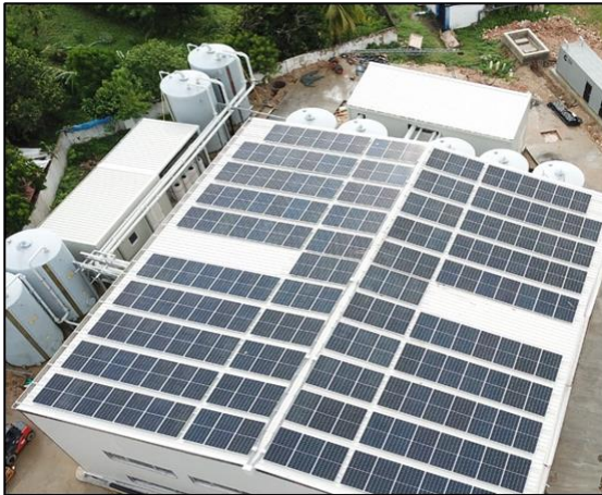
General view of the 50 L/s desalination plant
