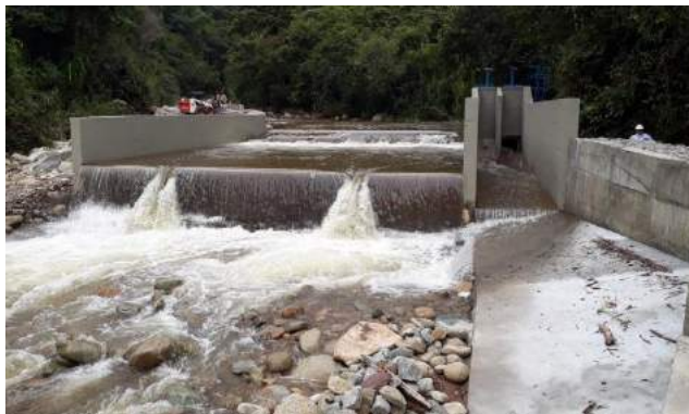
Aqueduct (Intake) - Socorro, Santander
