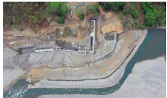
River protection Aqueduct - Mopal, Casanare
